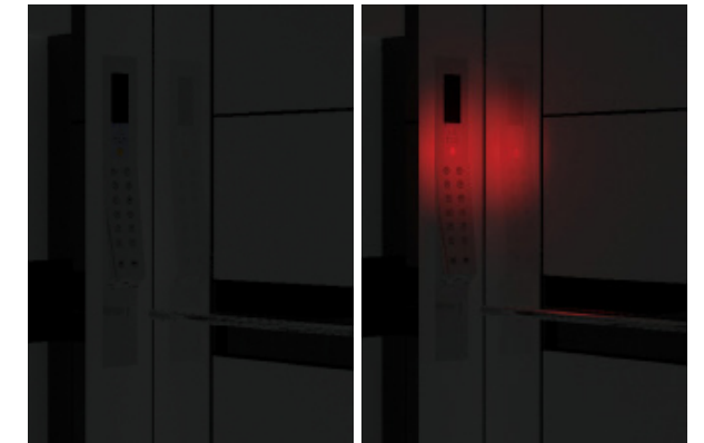
Without the emergency call button lighting for power outage
